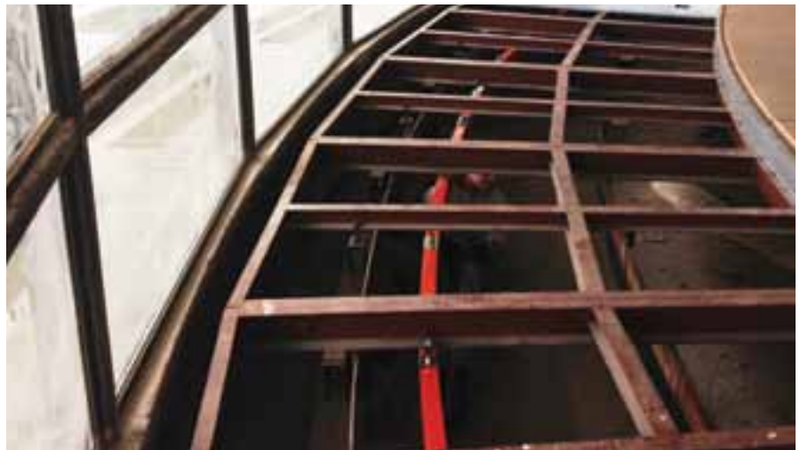
Exterior and interior of an enclosed track for rotating building motor
